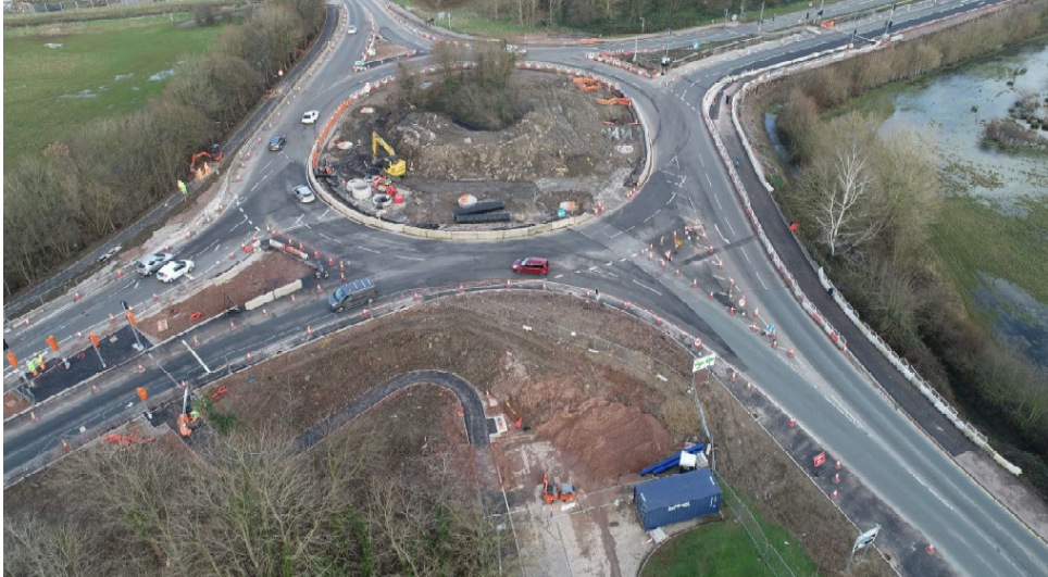
A40 West (North and South progress)
