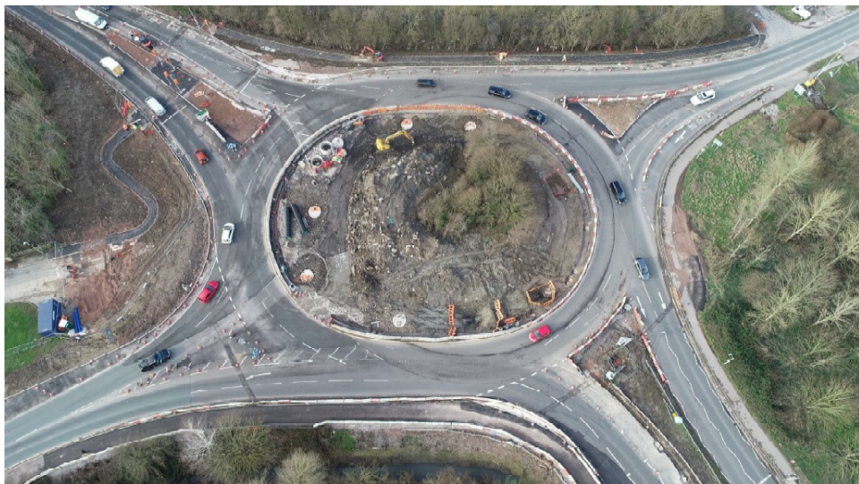
A40 Roundabout progress
