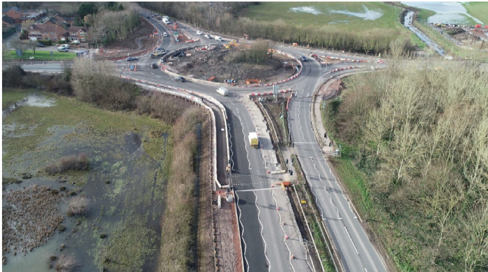
A40 East progress
